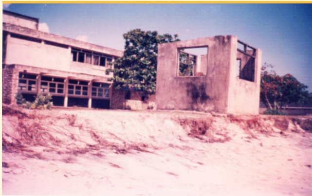
Radio-call house of KMFRTI as it appeared being threatened by the beach erosion in December 1995. ©Albogast T. Kamukuru
